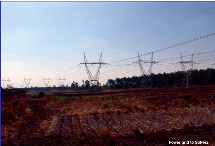
Power grid to Solwezi
