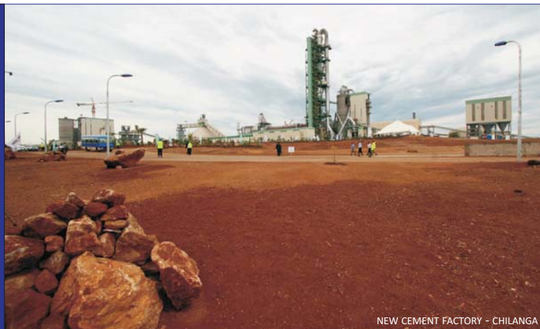
NEW CEMENT FACTORY - CHILANGA
