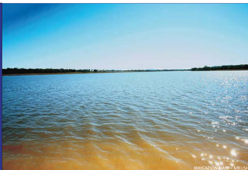
IRRIGATION DAM - MKUSHI
