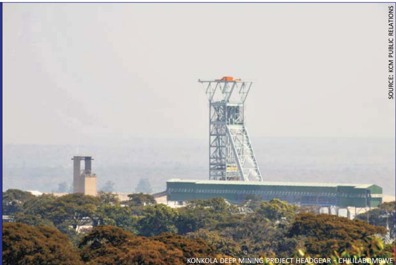
KONKOLA DEEP MINING PROJECT HEADGEAR - CHILILABOMBWE
